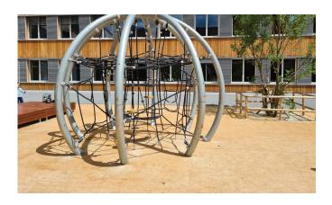
Matchwinner Velour is a sand dressed needlepunch surface which is available in 14 different colours, and designed to be inset into the surface making it ideal for education spaces to make the area bright and bold. Matchwinner Velour can be installed directly onto tarmac or equally with a Playrite shockpad to prolong the life and performance of the surface. Meets the EN15330 Part 2 standards.
