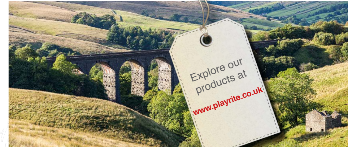
Dent Head Viaduct, Yorkshire Dales
