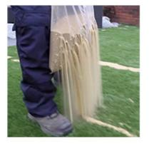
8. Apply sand to the installation, creating a natural finish and enhancing the durability of the turf.
