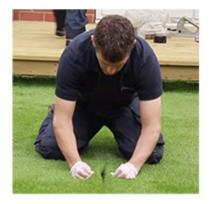
5. When placing two rolls together, pull as close as possible, and make sure the tufts are not caught in the seam.
