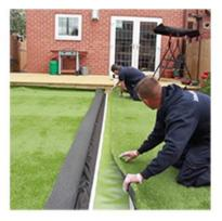
**6.** Trim any other excess and edges before laying your tape and glue as central as possible. Place the turf back over the adhesive..
