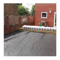
2. Lay a protective undersheet on the base. This acts as a barrier to weeds and protects the grass from sharp stones.
