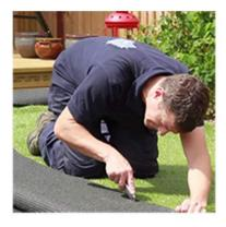
**4.** Use a sharp Stanley knife to trim down according to the shape of the area. You can also trim further excess once the turf is fixed..
