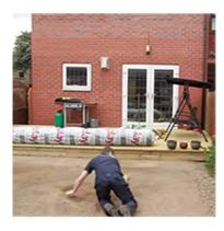
1. Once you've removed existing turf fill the area with sand. Spread, level and compact to create a sturdy level base.
